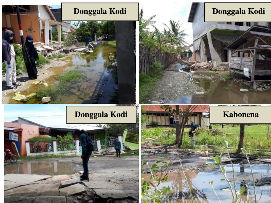
Figure 6 Puddles that are thought to have originated from the subsurface at several locations along the fault line
