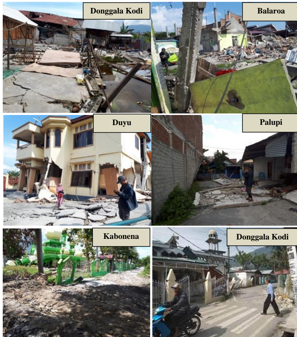
Figure 3 Buildings damaged by surface rupture, which are exactly located on the active Palu-Koro fault line
