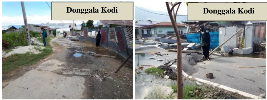
Figure 4 The road has meanders, and the road asphalt slopes upwards due to the buildup of frictional forces from displacement faults
