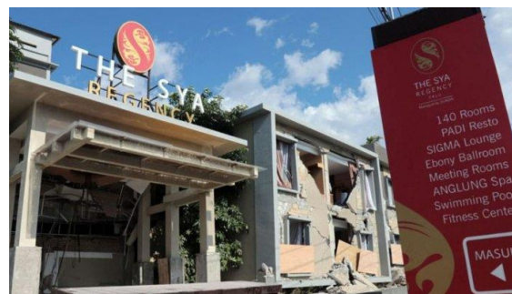
Fig 2. The Sya Regency Hotel Post Earthquake
